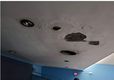
Figures 9 and 10: Peeling ceiling in the balcony, likely caused by moisture damage from the roof.
