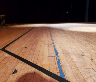
Figure 22: Professionally sand down and refinish existing floor $2-3/SF
