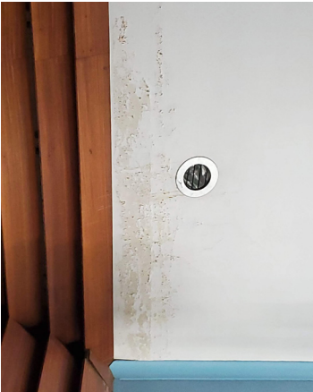
Figure 11: Ceiling damage near the stage
