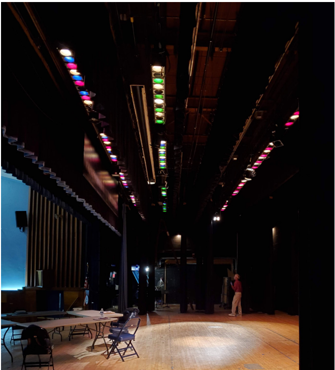
Figure 35: The strip lights shown here are very inefficient and don't provide much flexibility. It is recommended to eventually phase these out in favor of more adjustable and movable options.
