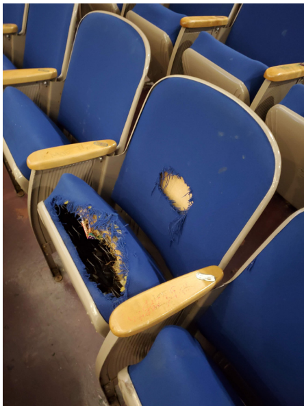
Figure 7: Seats that are damaged this badly need to be reupholstered or replaced.
