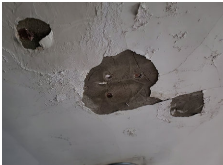
Figures 9 and 10: Peeling ceiling in the balcony, likely caused by moisture damage from the roof.
