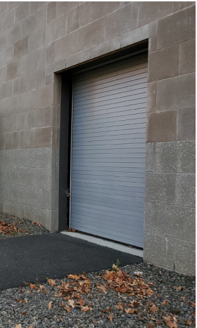
Figure 21: On the left is an image of the loading doors at Poughkeepsie High School. On the right is the roll-up door we saw at Rhinebeck High School. As the Poughkeepsie auditorium only has one set of loading doors, it is recommended that they be upgraded to a roll-up door.
