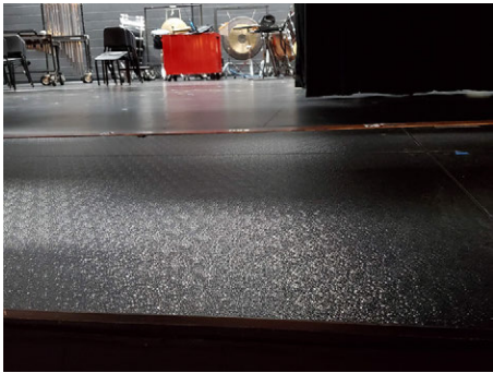
▲ Black RFP covers the proscenium extension – this material is not recommended as it is slippery.
